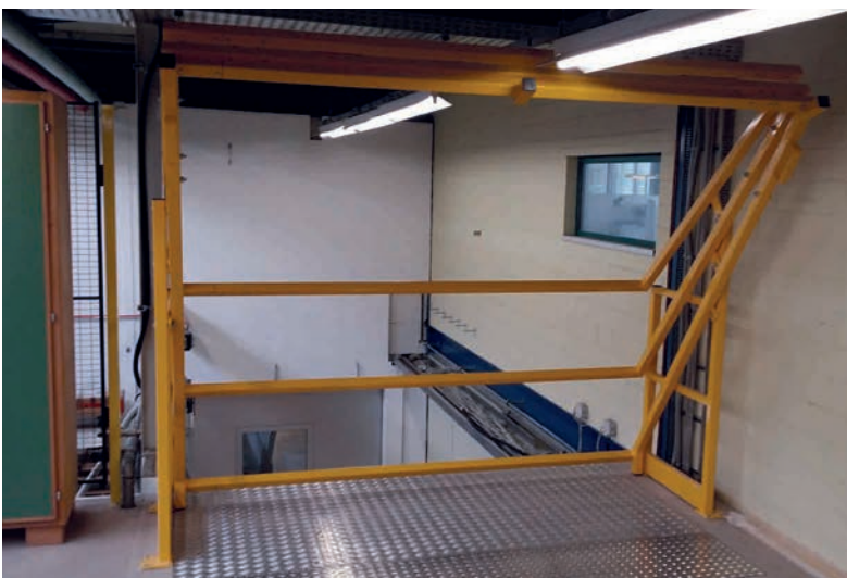
Storage platform with rocker and safety gate
